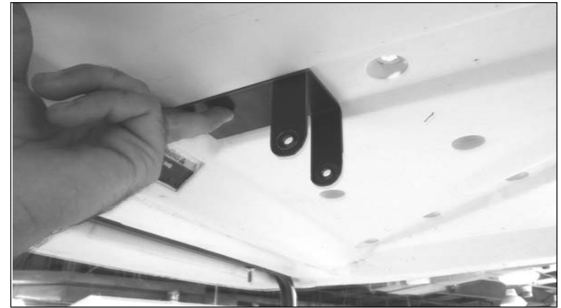
Figure 2 - Mount Bracket Installation
